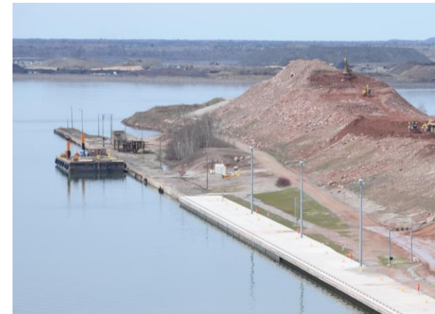
Western Limit of completed North Upstream Approach Wall Work (30 APR 2025)
